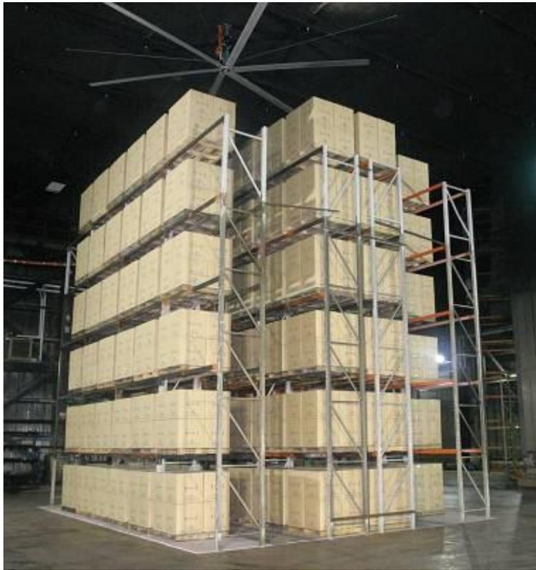
**Figure 4-3: Typical rack storage array of standard plastic commodity**
