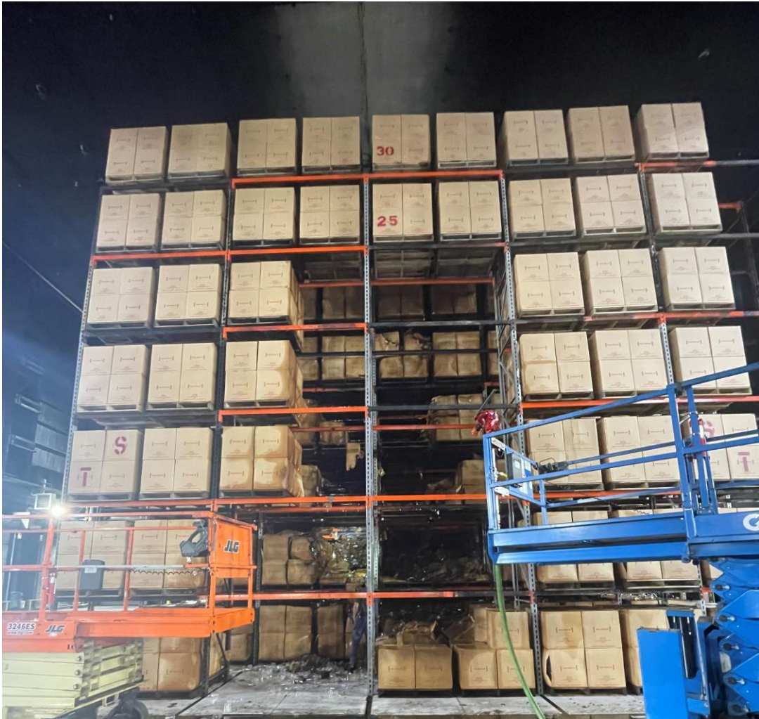
Figure 3-18: Images taken after test for damage assessment of Test LS-5
