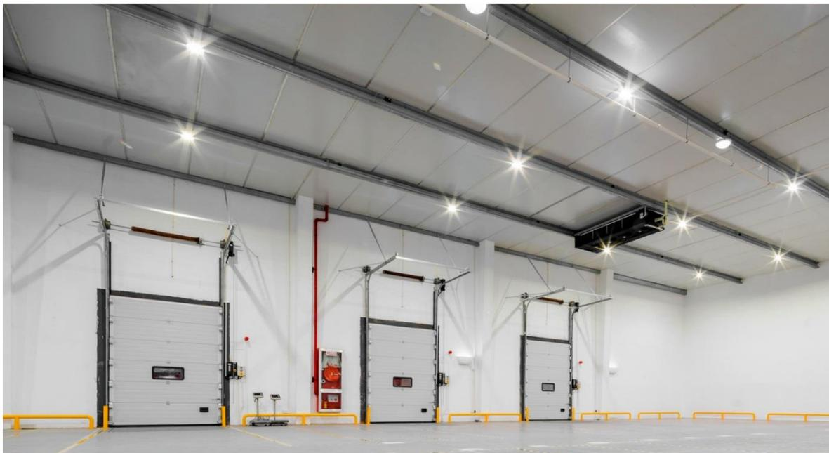
(b) Insulation present below the ceiling reduces the purlin channel depth [4]
