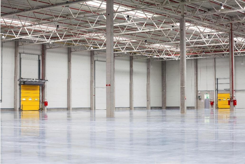
(a) Truss structures present below the ceiling (unobstructed ceiling) [5]
