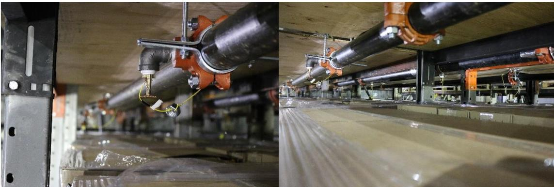
Figure 3.4.1-5: Photos of in-rack sprinkler placement – Test 3.
