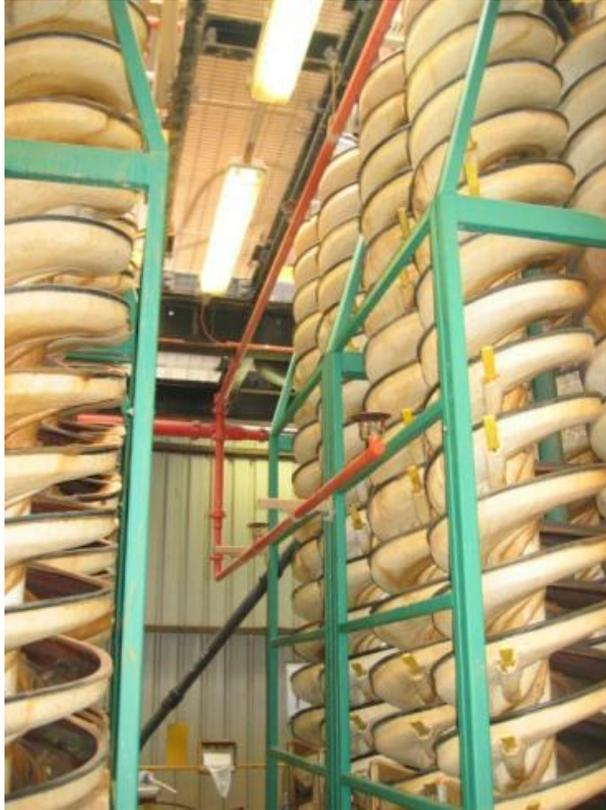
Figure 1-3: Example of protection for spiral separators in a mining operation. The sprinklers are hung in the middle of the aisle.
