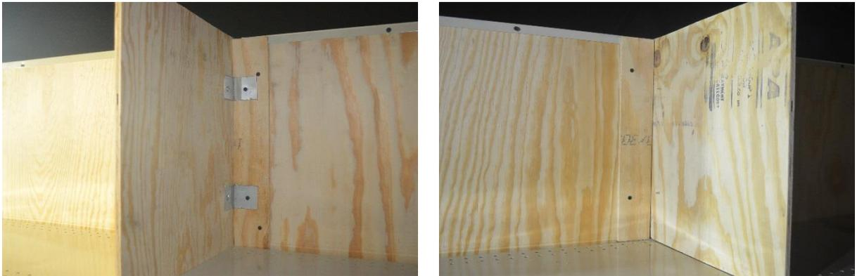
Figure 2-10: Construction of lateral flame break (penetrations at shelving upright covered by sheet of flame break material).
