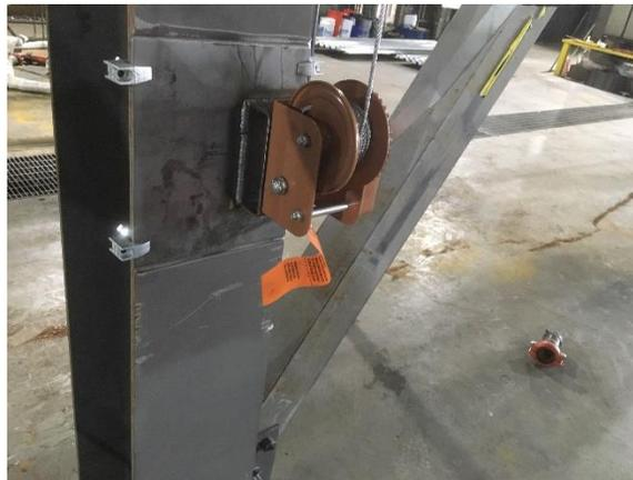
Figure 2-5: Crankshaft for smoke vent activation.
