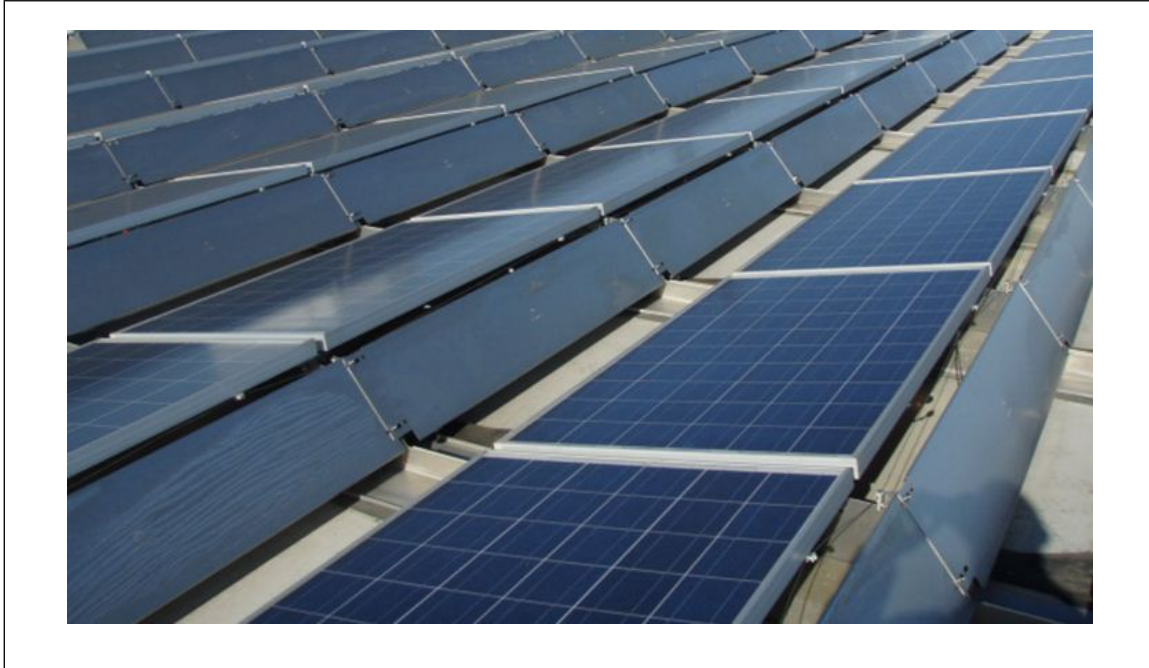
Fig. 2.1.2-1. Wind deflectors provided on the high sides of panels in each row (closed array)
