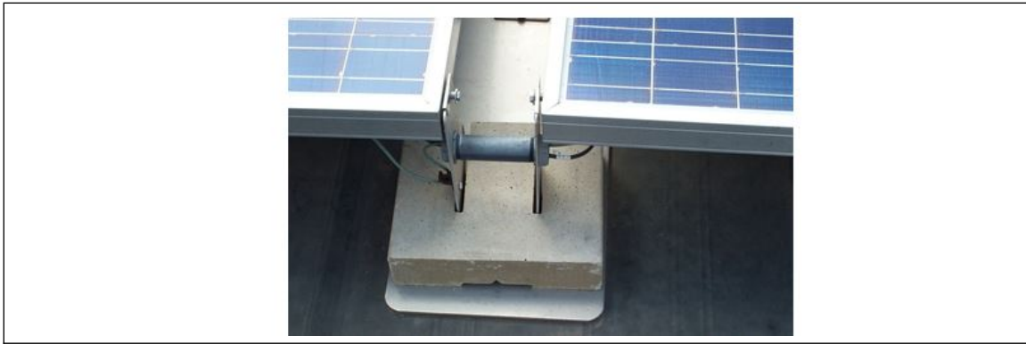
Fig. 2.1.2.4.2-1. Slotted pedestal
