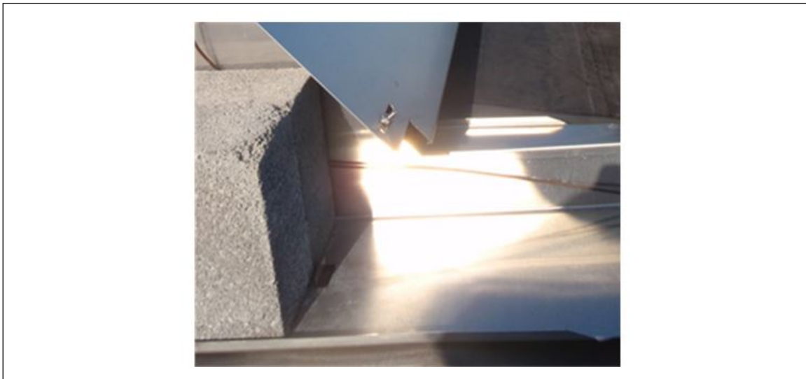
Fig. 2.1.2.4.2-2. Flanged pedestal
