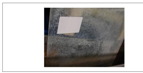
Fig. 3.2.1-4. Weathered greenhouse roof glass panel
