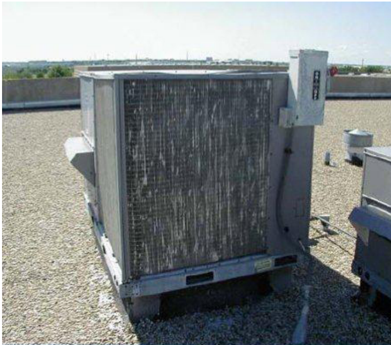
Fig. 3.3.1-1. Hail damaged HVAC unit
