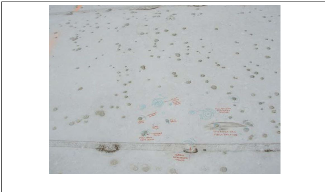
Fig. 3.5.2-1. Hail damage to 15-year old single-ply membrane
