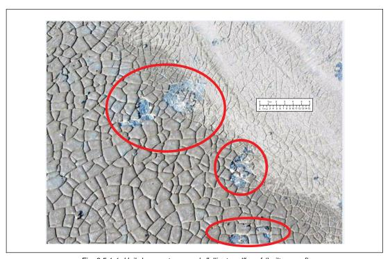
Fig. 3.5.1-1. Hail damage to severely "alligatored" roof (built-up roof)
