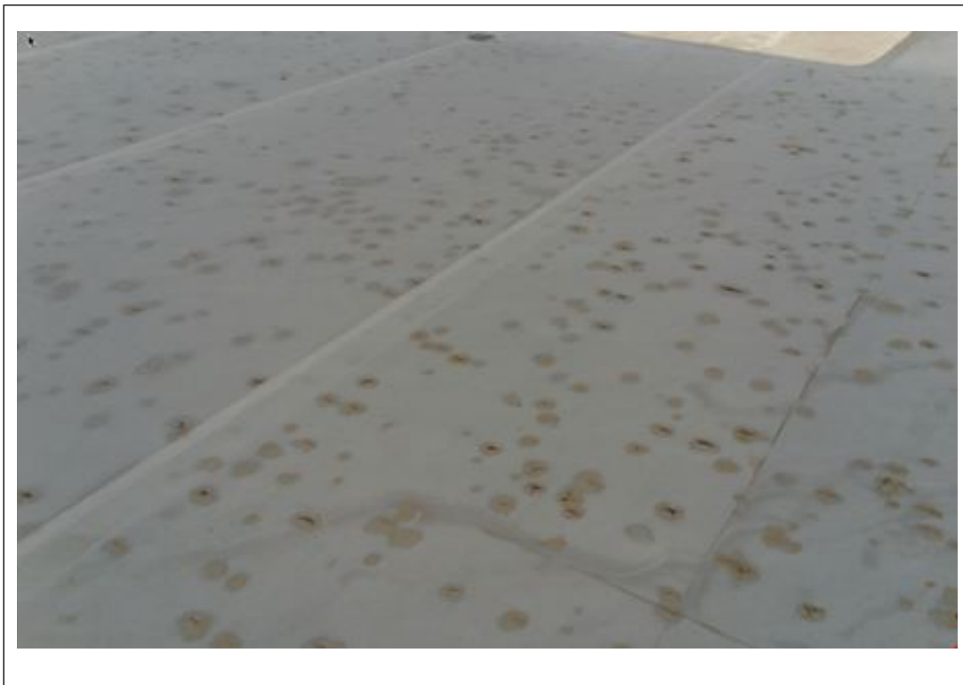
Fig. 3.1.1-1. Single-ply membrane roof 0.045 in. (1.1 mm) thick cut by hail
