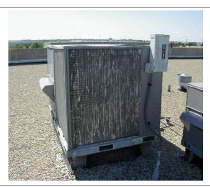
Fig. 3.3.1-1. Hail damaged HVAC unit
