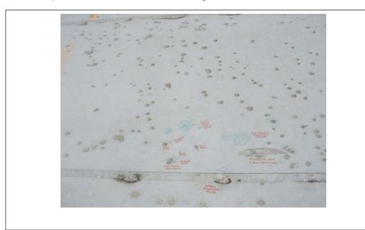
Fig. 3.5.2-1. Hail damage to 15-year old single-ply membrane
