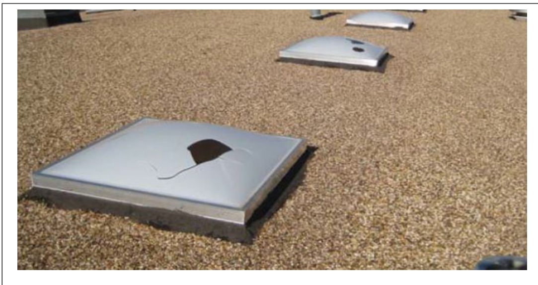
Fig. 3.2.1-1. Holes in acrylic skylights caused by hail
