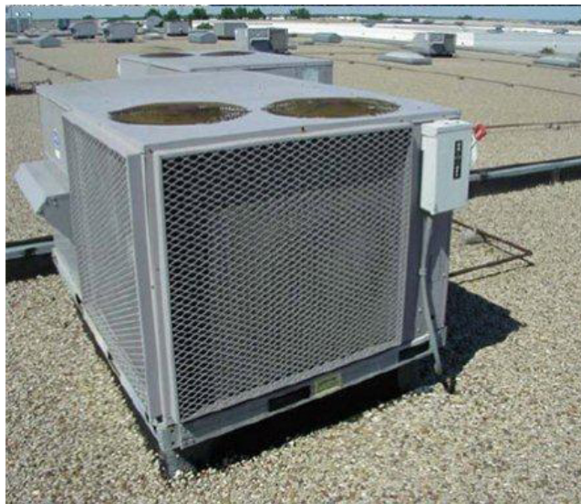
Fig. 3.3.1-2. HVAC unit with hail guard over condenser cooling fins at same location as hail damaged unit in Figure 3.3.1-1
