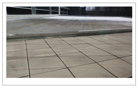
Fig. 3.1.1-4. Concrete paver covered roof
