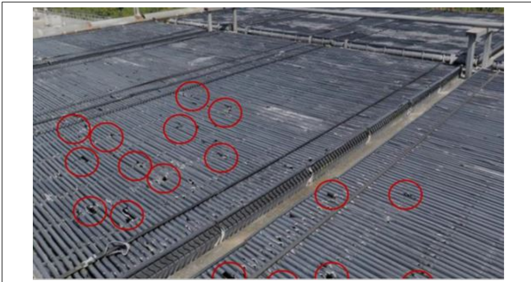
Fig. 3.4.1-2. Hail damage to plastic drift eliminators
