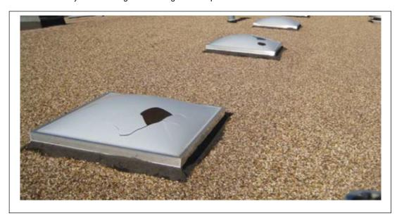
Fig. 3.2.1-1. Holes in acrylic skylights caused by hail
