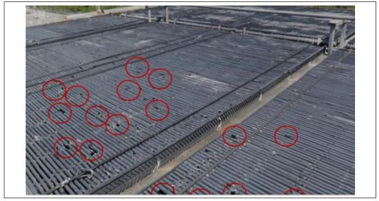
Fig. 3.4.1-2. Hail damage to plastic drift eliminators
