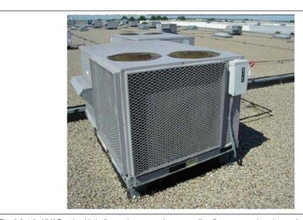
Fig. 3.3.1-2. HVAC unit with hail guard over condenser cooling fins at same location as hail damaged unit in Figure 3.3.1-1
