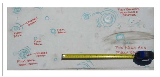
Fig. 3.5.2-2. Close-up of hail damage in Figure 3.5.2-1
