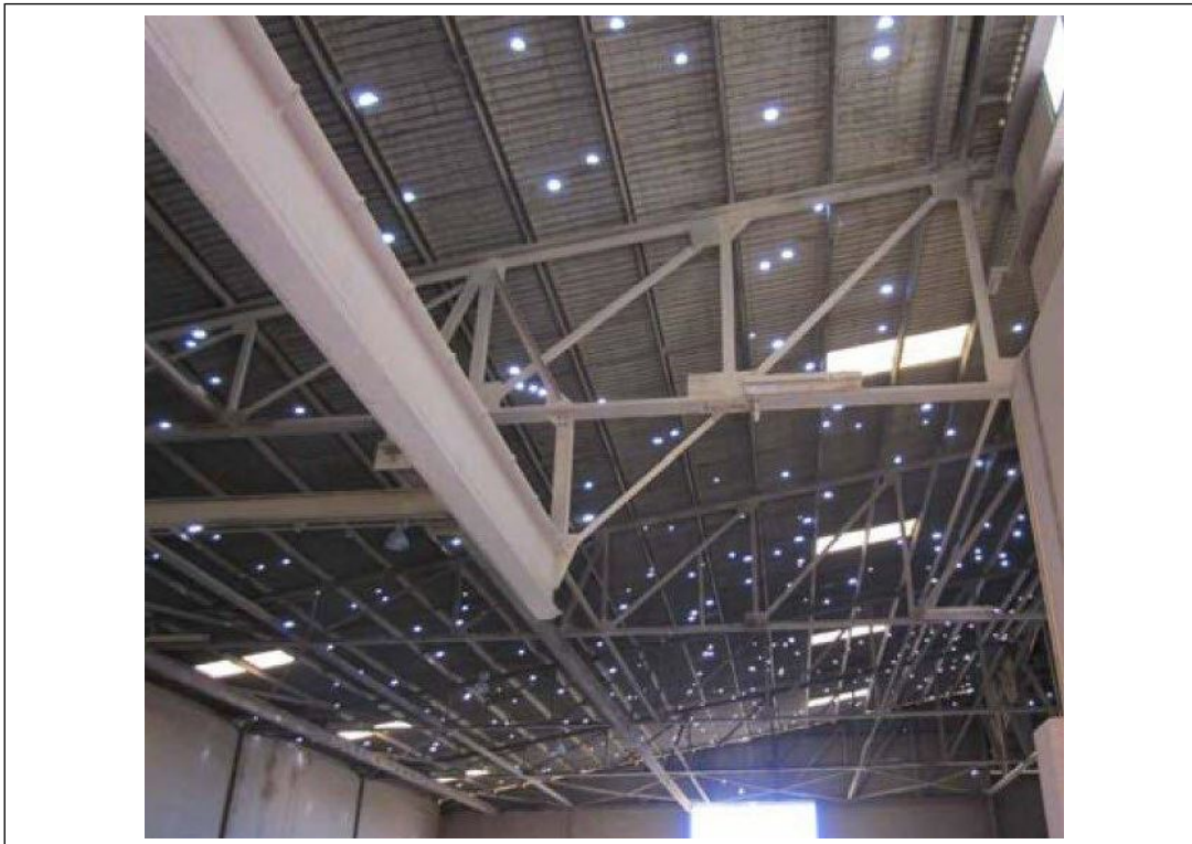
Fig. 3.8-1. Hail damage to asbestos cement roof
