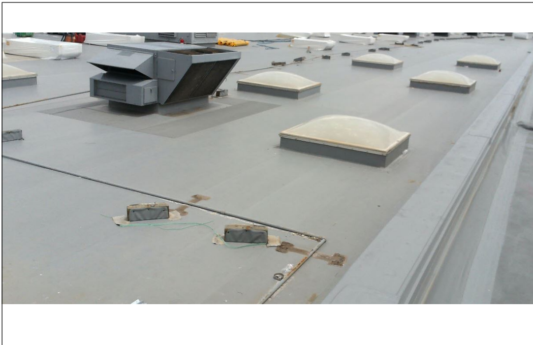
Fig. 3.1.1-3. Undamaged single-ply membrane roof cover adjacent to damaged roof in Figures 3.1.1-1 and 3.1.1-2
