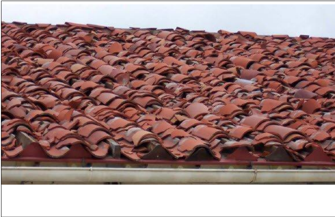
Fig. 3.8-2. Hail damage to clay roof tiles
