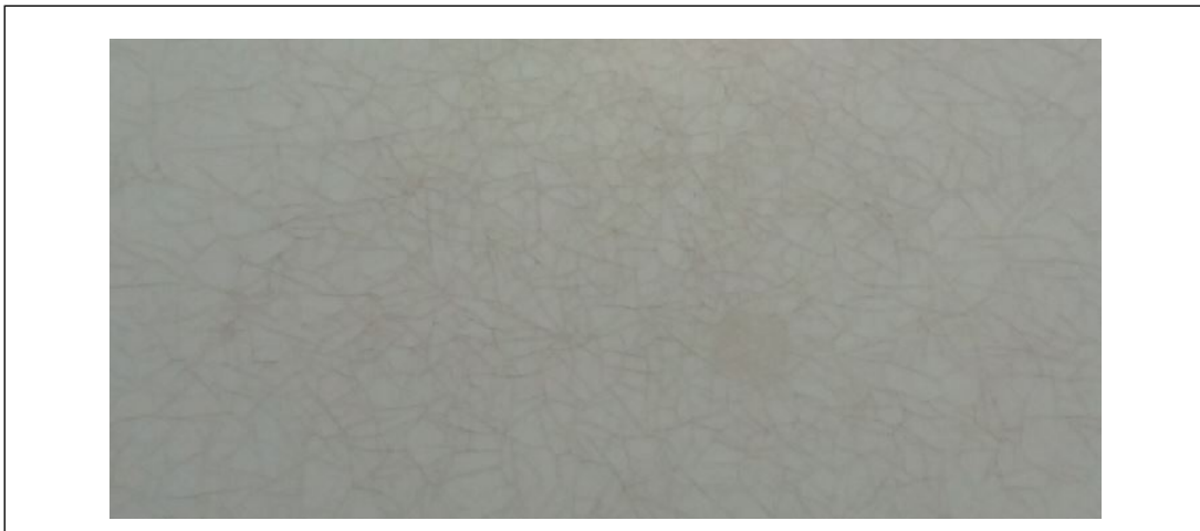
Fig. 3.2.1-3. Close up of embrittled acrylic skylight in Fig. 3.2.1-2
