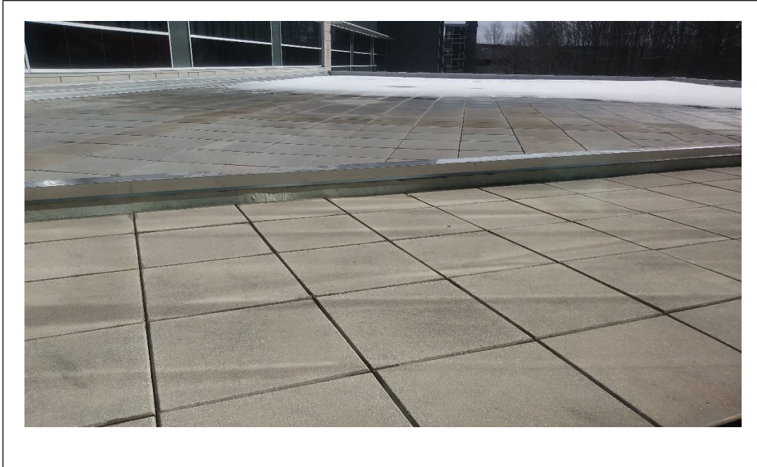
Fig. 3.1.1-4. Concrete paver covered roof
