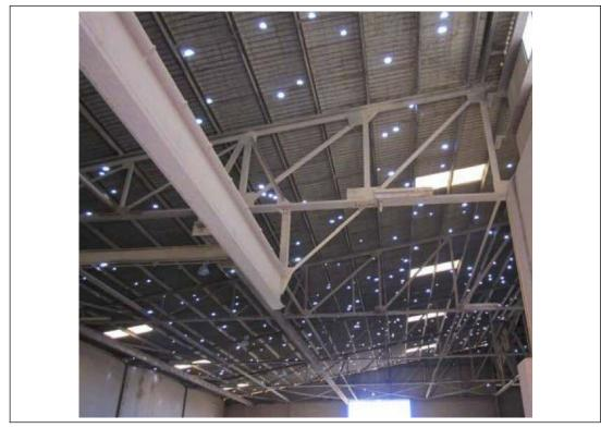
Fig. 3.8-1. Hail damage to asbestos cement roof
