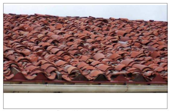
Fig. 3.8-2. Hail damage to clay roof tiles
