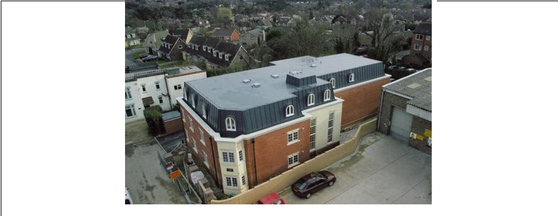
Fig. 2. Steep sloped mansard roof
