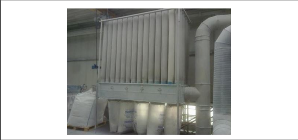
Fig. 3.4.1.1-1. Example of an enclosureless collector
