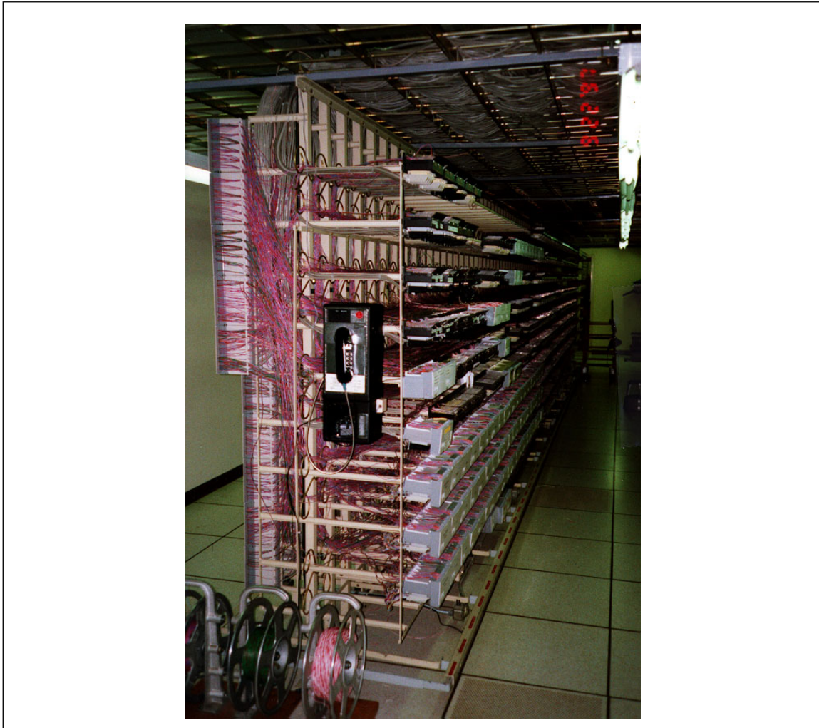
Fig. 8. Main distribution frame (MDF)
