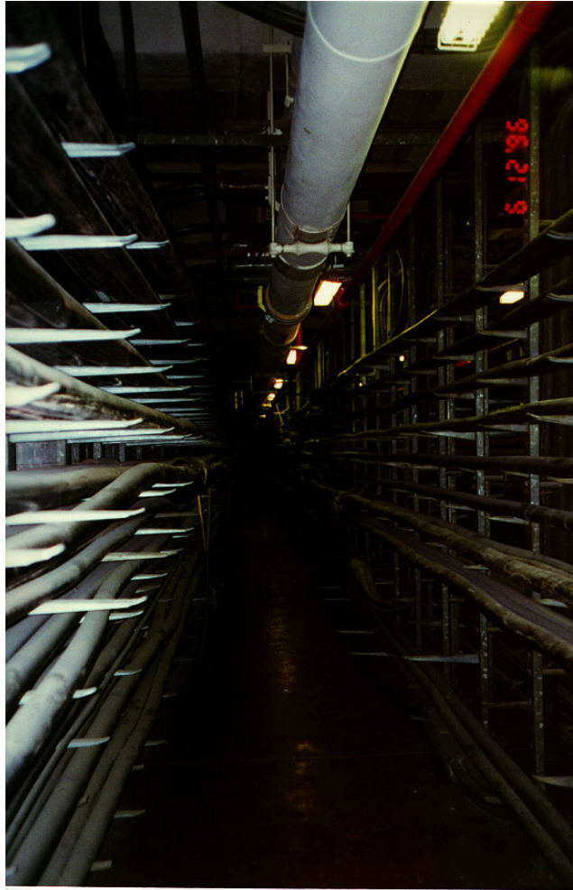
Fig. 7. Cable vault located in a large metropolitan switching center
