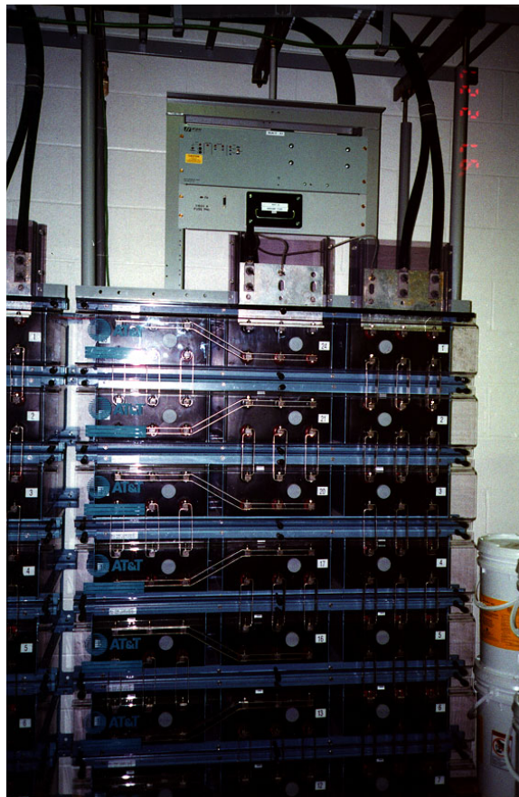
Fig. 10. Valve-regulated lead acid batteries
