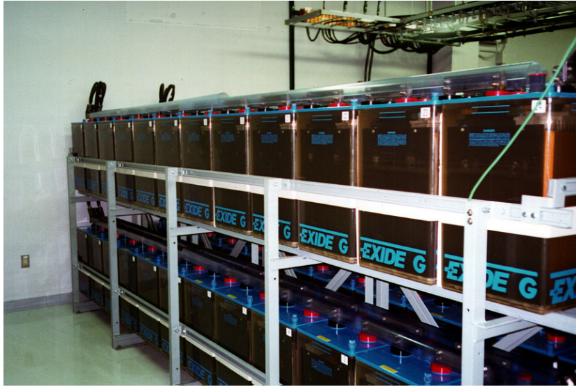
Fig. 9. Flooded-cell battery room
