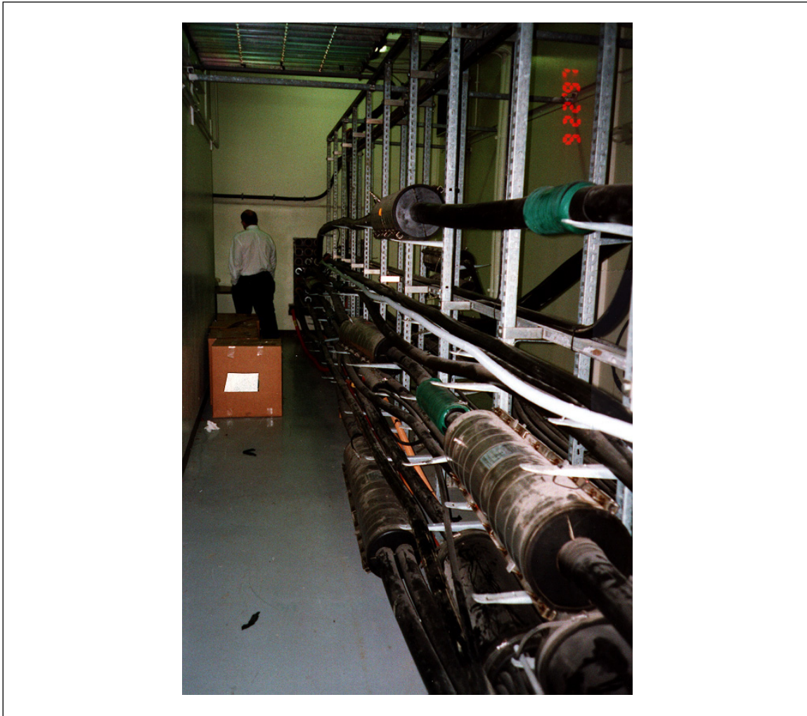
Fig. 6. Cable tunnel for an end office
