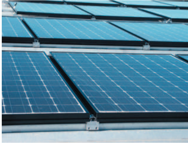
Fig. 3.2.2-1. Solar panels secured to standing seam roofs using external seam clamps
