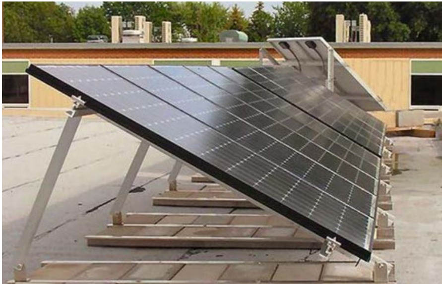
Fig. 3.2.1.1-2. Solar panels with steeper slopes or lacking wind deflectors will experience greater wind effects
