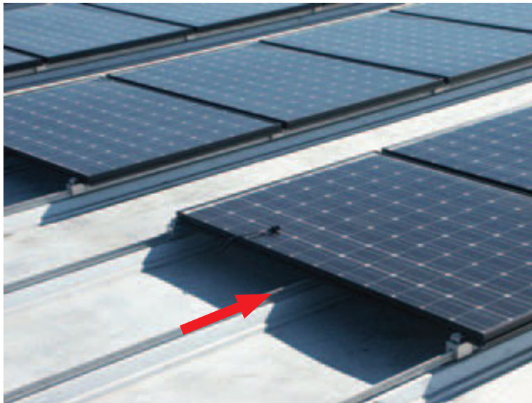
Fig. 3.2.2-2. Unacceptable arrangement unless specifically tested and FM Approved: clamp missing from SSR rib below middle of outer panel edge
