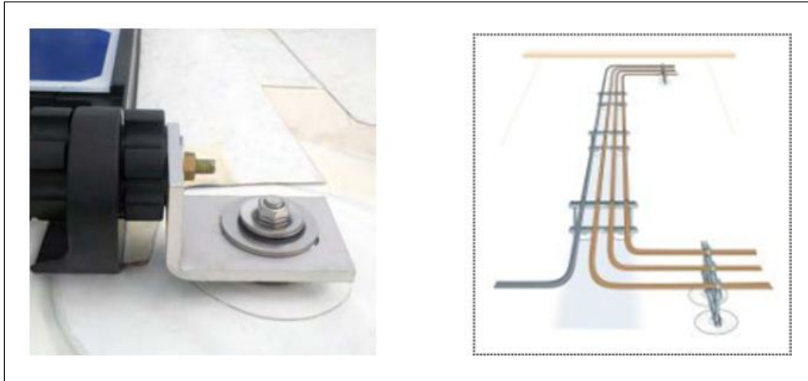
Fig. 2.1.1.9-1a and b. Examples of mechanical anchors used to secure equipment to the roof deck or roof framing
