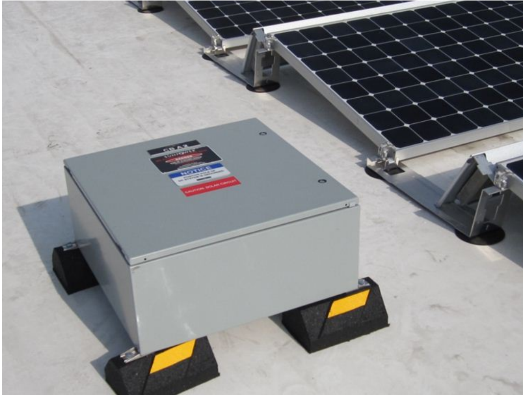
Fig. 3.2.1.1-3. Equipment lacking anchorage to roof framing
