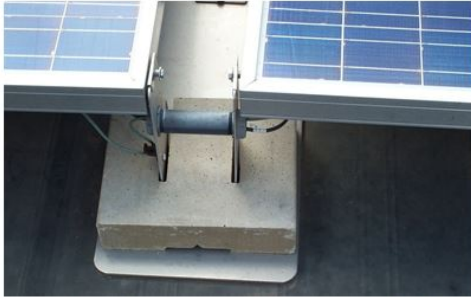
Fig. 2.1.1.11-1. Slotted pedestal
