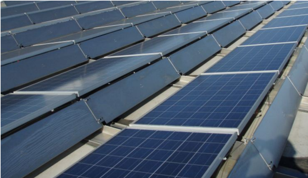
Fig. 2.1.1.1-1. Wind deflectors provided on the high sides of panels in each row (closed array)
