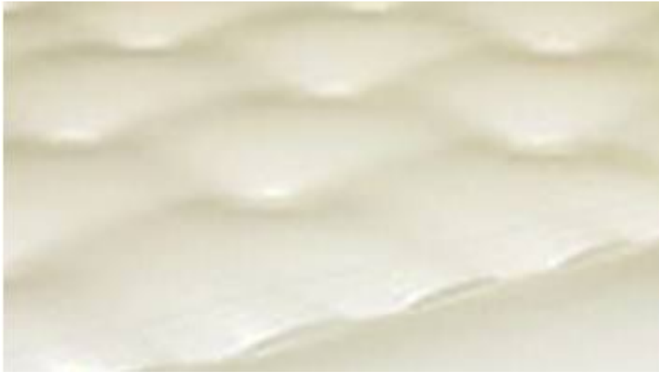
Fig. 3.2.1.1-1. Mechanically fastened roof cover billowing when subjected to wind pressure
