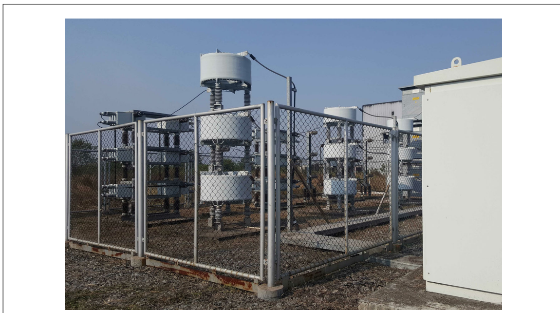
Fig. C.5.1-4. Capacitors, reactors and filters for a static reactive compensator system
