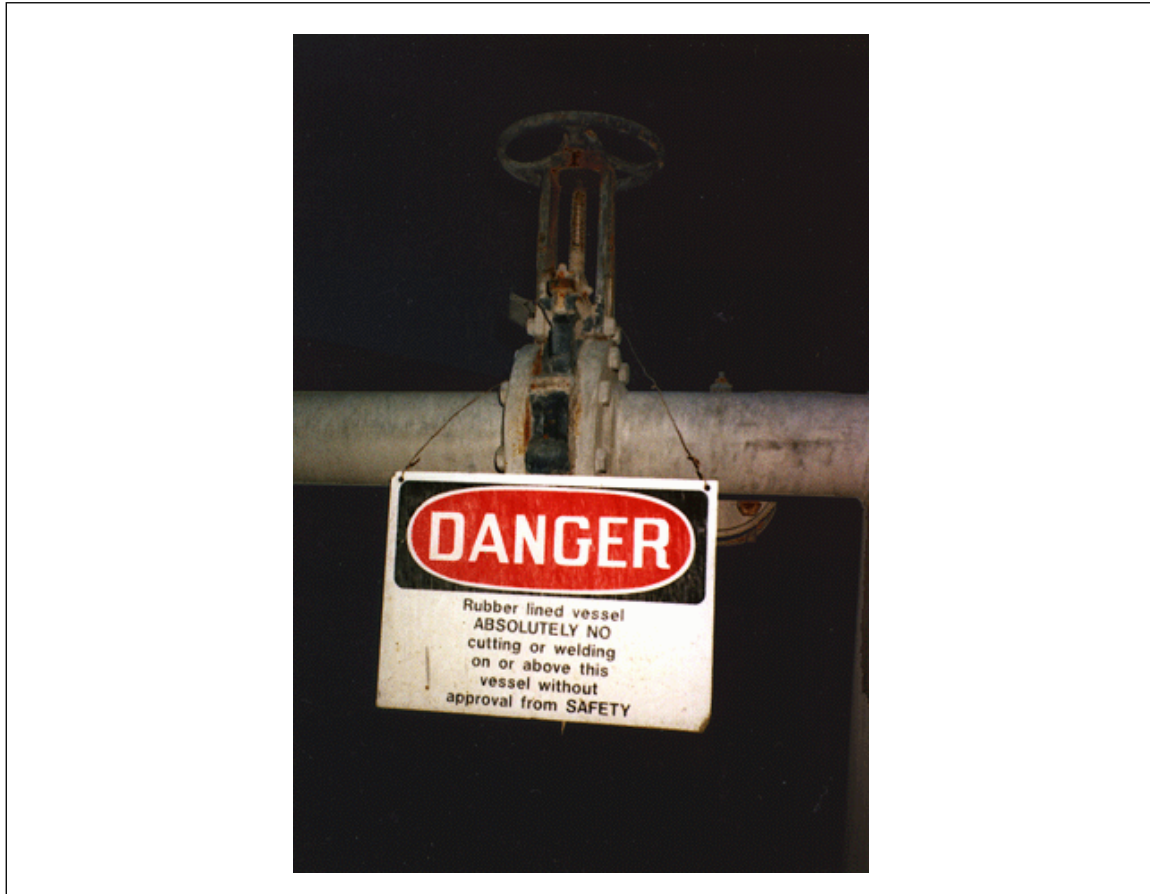
Fig. 9. Signage indicating a rubber-lined vessel below
