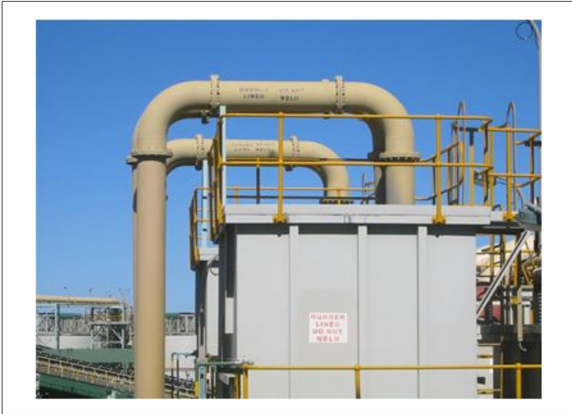
Fig. 8. Label warning of rubber-lined equipment including piping
