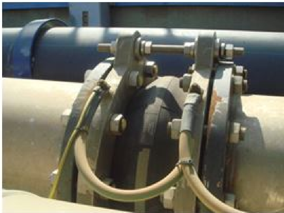
Fig. 22. Flexible steel connection
