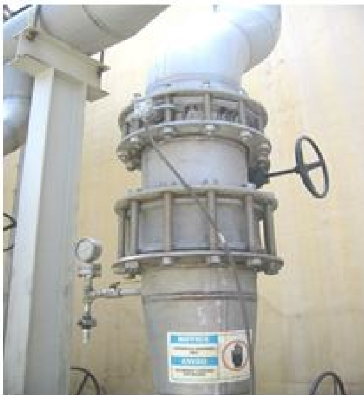
Fig. 20. Flexible steel connection
