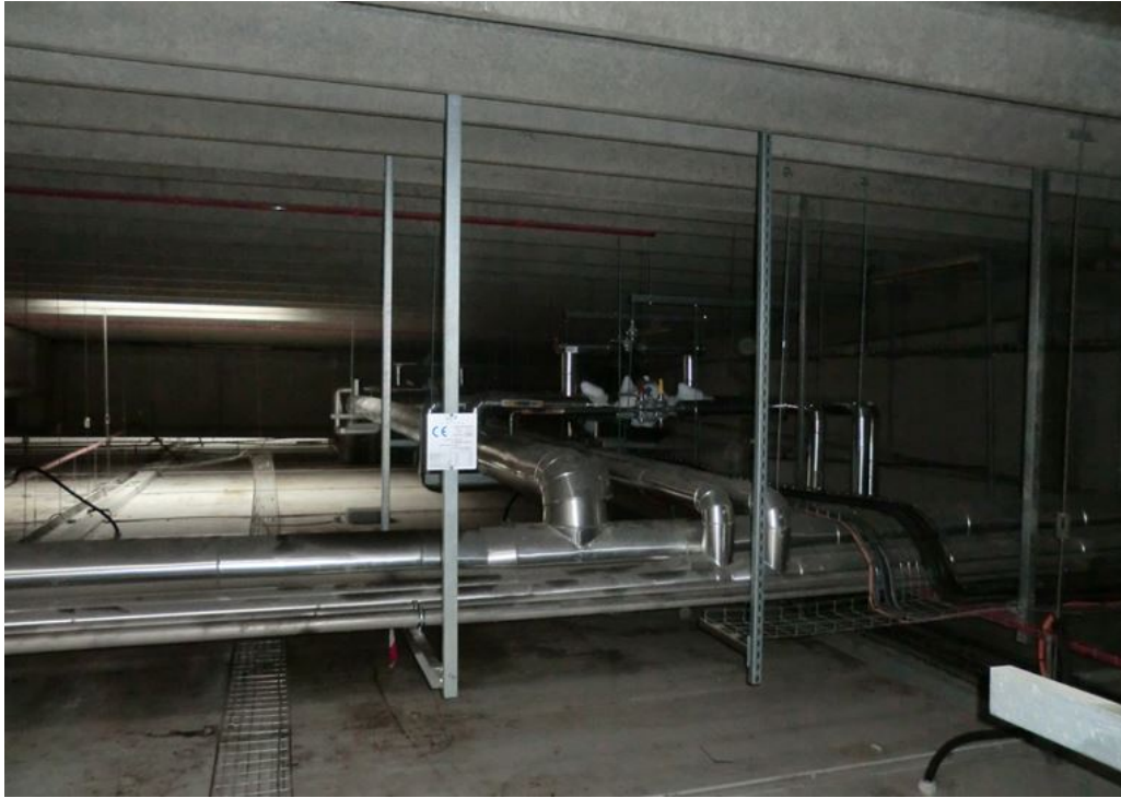
Fig. 1. Refrigerant piping
