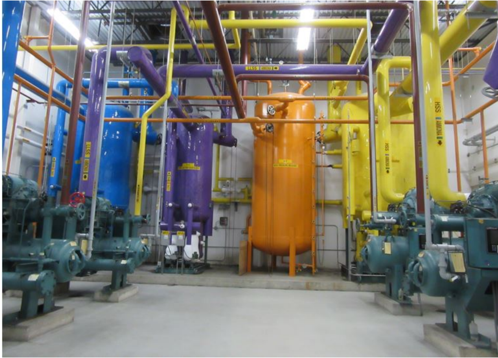
Fig. 6. Direct refrigeration system machinery room
