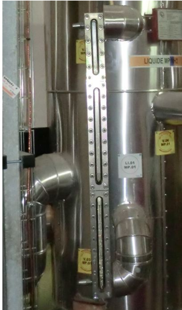
Fig. 3. Typical armored gauge glass assembly
