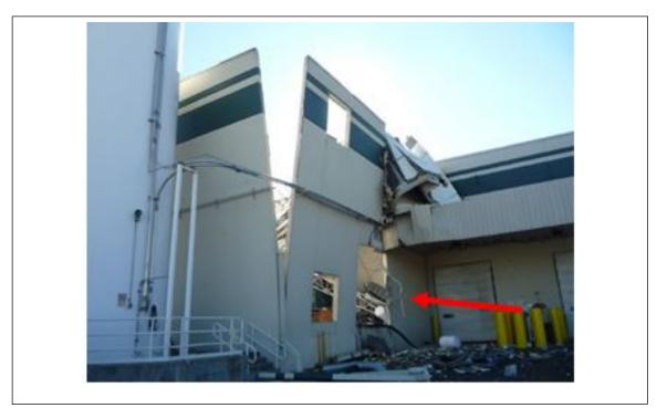
Fig. 10. The boiler building showing the rear walls; the red arrow shows the area where the deaerator exited the building
