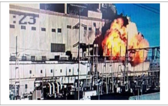
Fig. 24. Deflagration fireball erupting from the silo enclosurecollapsed feeder deck
