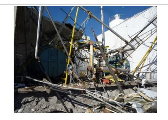
Fig. 11. The boiler room, showing the two front walls completely blown to the ground
