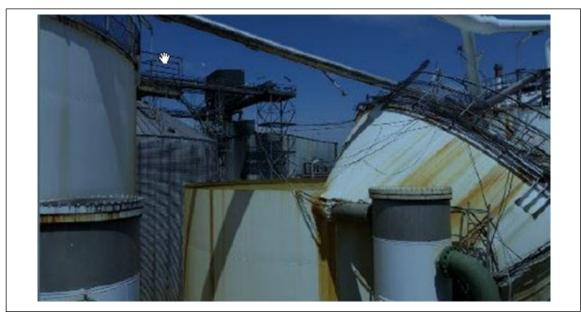
Fig. 22. Upper portion of fermenter after failure
