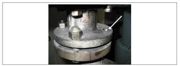
Fig. 3. Bolted connection on pressure vessel pressure boundary showing missing bolt
