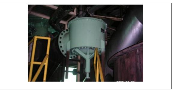
Fig. 4. Eighteen in. (450 mm) diameter, weighted pallet vacuum relief valve (set pressure on order of inches of water [mm of water] with relief capacity on order of 20,000 scfm [566 m<sup>2</sup>/min] air)
