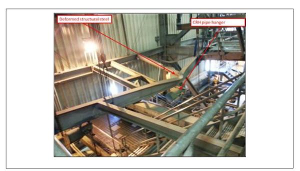
Fig. 17. Damage to the structural steel due to pipe movement
