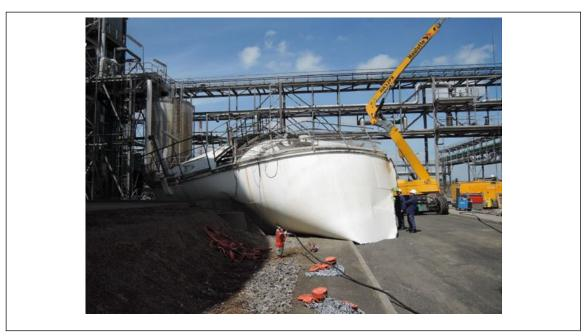
Fig. 23. The roof of the fermenter after failure
