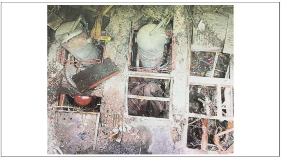
Fig. 18. Damage due to heat exchanger failure
