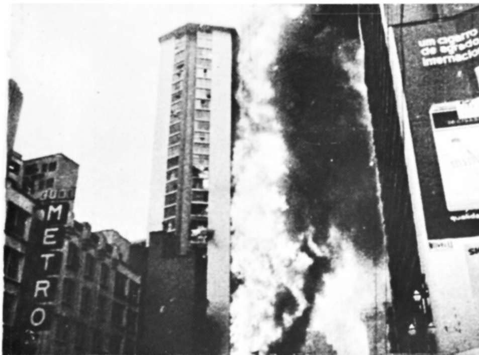
Fig. 10. Exterior fire spread in a high-rise building, as well as severe fire exposure to adjacent building
