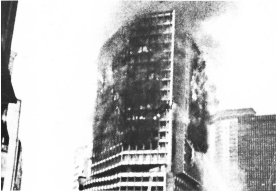
Fig. 7. Exterior fire spread in a high-rise building
