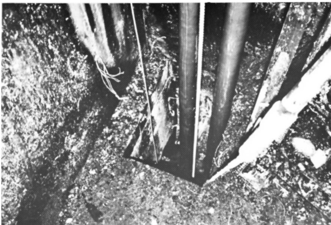
Fig. 11. Hole through floor slab in telephone closet allowed fire spread to the upper floors; these holes, approximately 12 by 18 in. (300 by 450 mm), were not fire stopped
