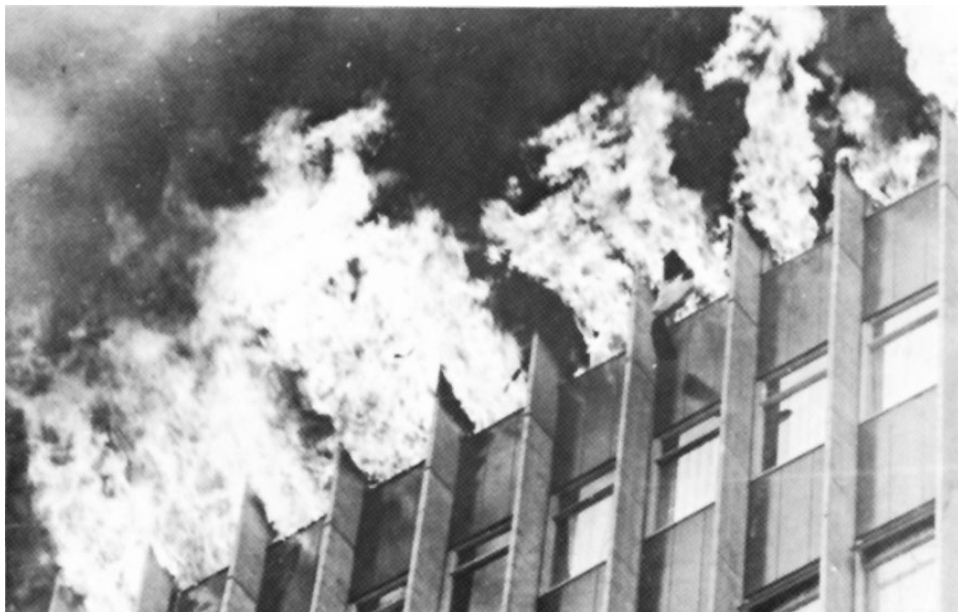
Fig. 8. Exterior fire spread in a high-rise building
