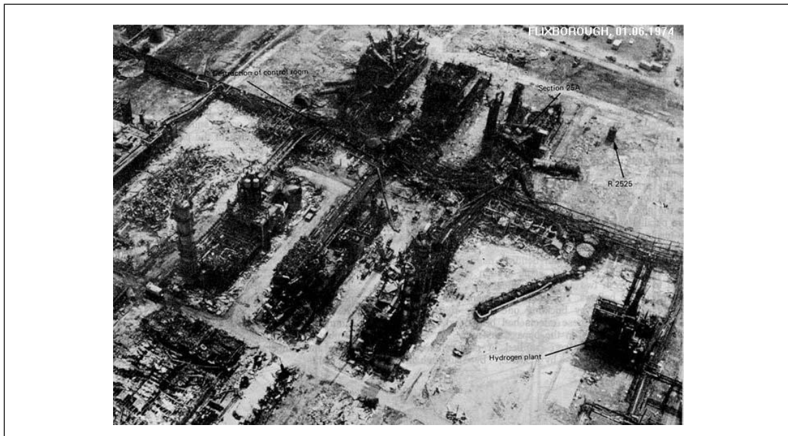
Fig. 7. Process area damage at Flixborough
