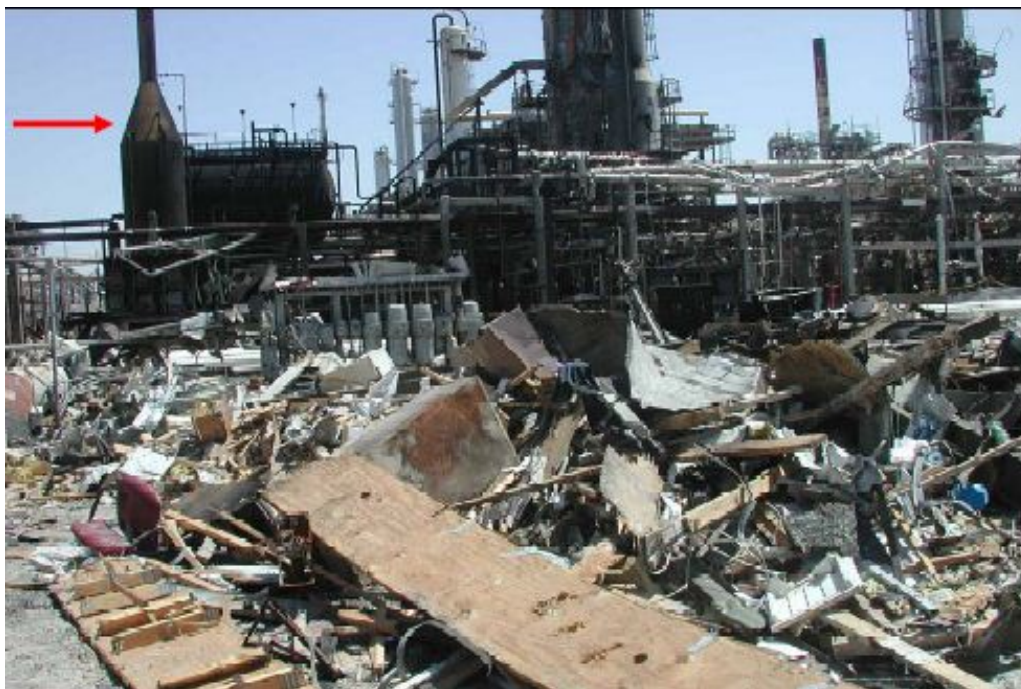
Fig. 10. Blow-down drum at BP, Texas City (photo from the U.S. CSB final report)
