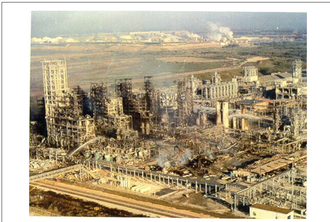
Fig. 9. Damage to Phillips plant following the VCE
