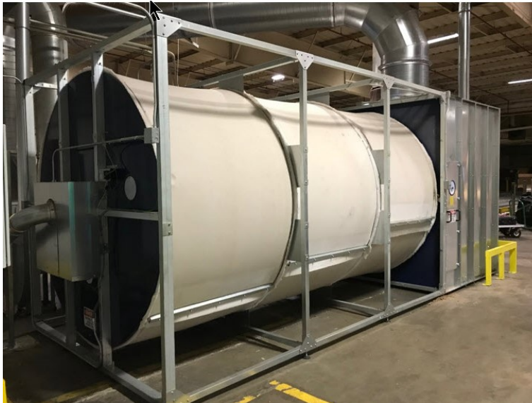
Fig. 3.4.1.2-1. Example of an enclosureless drum filter
