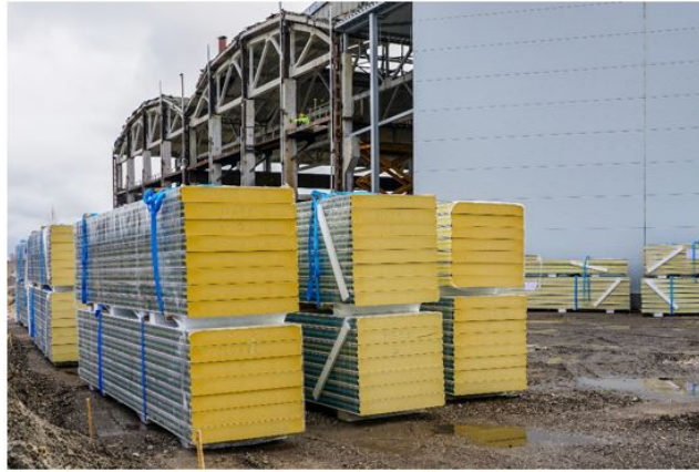
Fig. 3.2.1.1-1. Polyurethane foam core example (usually a yellow color)
