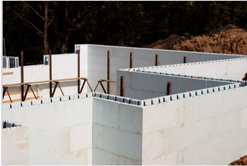
Fig. 3.2.23-1. Insulated concrete form (made from EPS/XPS foam blocks)
