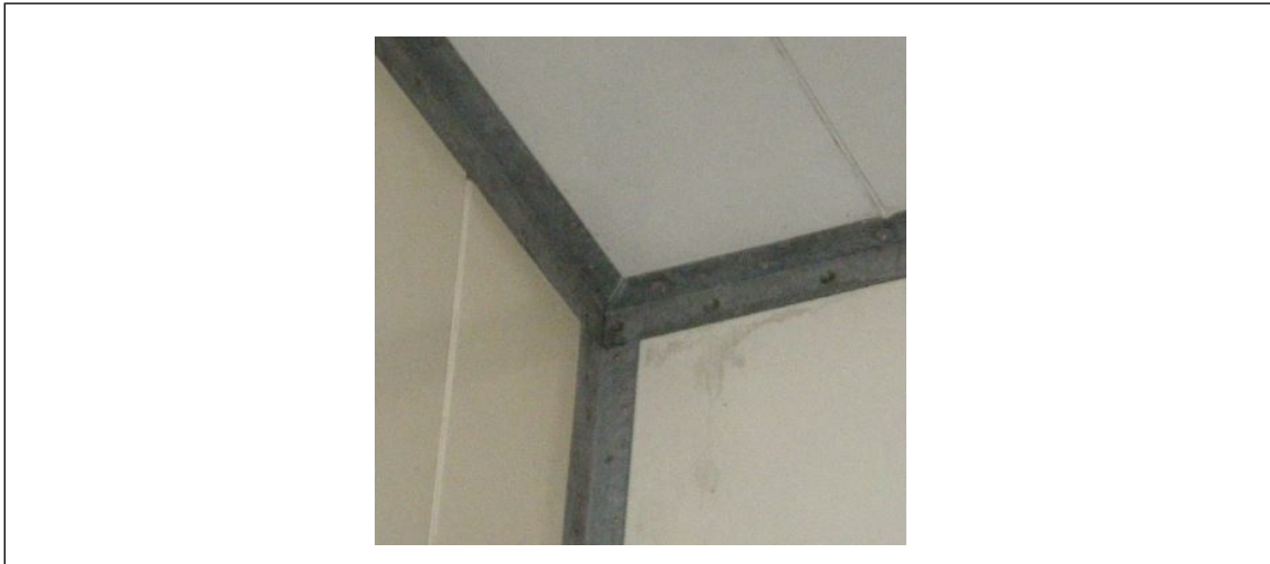
Fig. 2.2-1. Angles provided for securement
