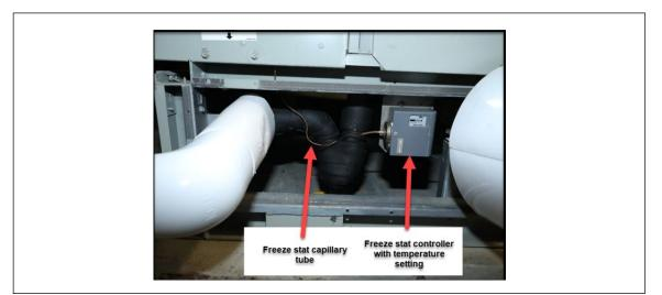
Fig. 3.5-3. Freeze stat controller and capillary tube with cover plate removed
