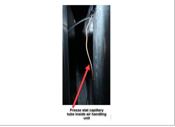
Fig. 3.5-4. Continuation of the freeze stat's copper capillary tube inside the air handler
