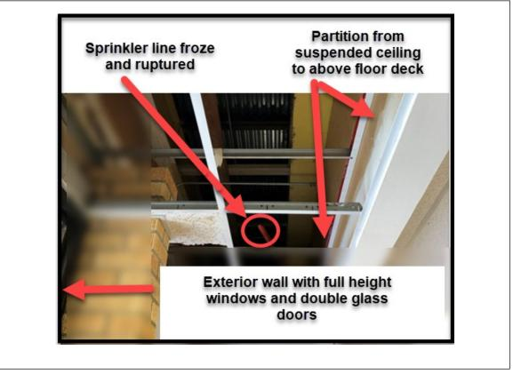
Fig. 3.4-1. Frozen/ruptured sprinkler line above suspended ceiling
