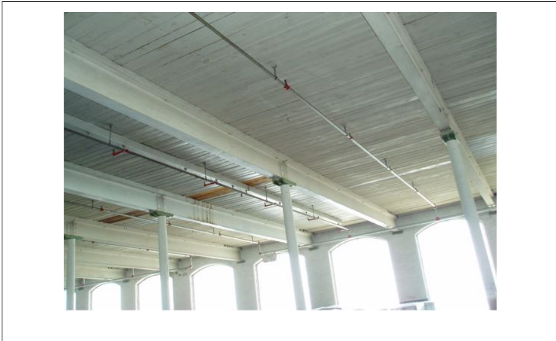
Fig. 1.1-3. Typical plank-on-steel building
