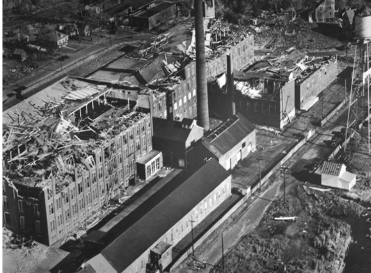
Fig. 3.2-1. Plank-on-timber textile mill in Pawcatuck, CT damaged by the 1938 hurricane
