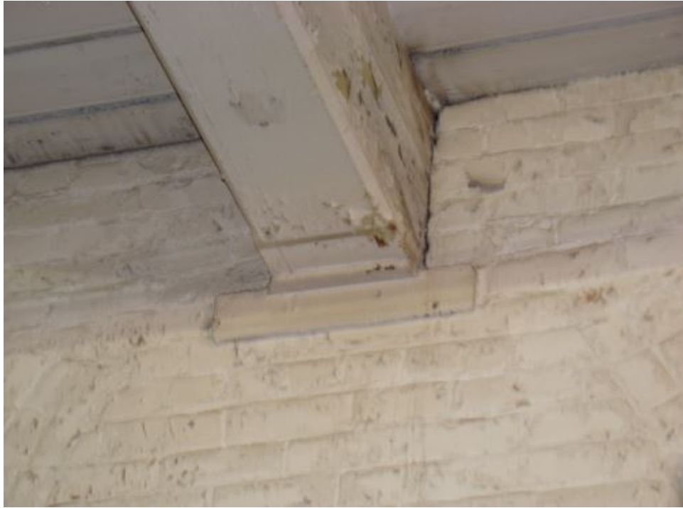
Fig. 3.1-4. Wood roof beam rests on metal plate in brick wall
