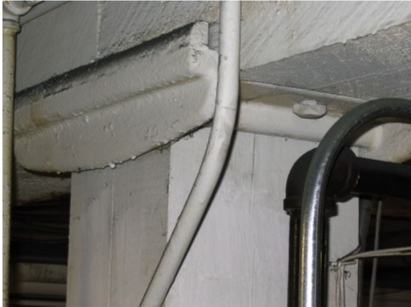
Fig. 3.1-2. Closeup of wood roof beam resting on wood column with metal column cap
