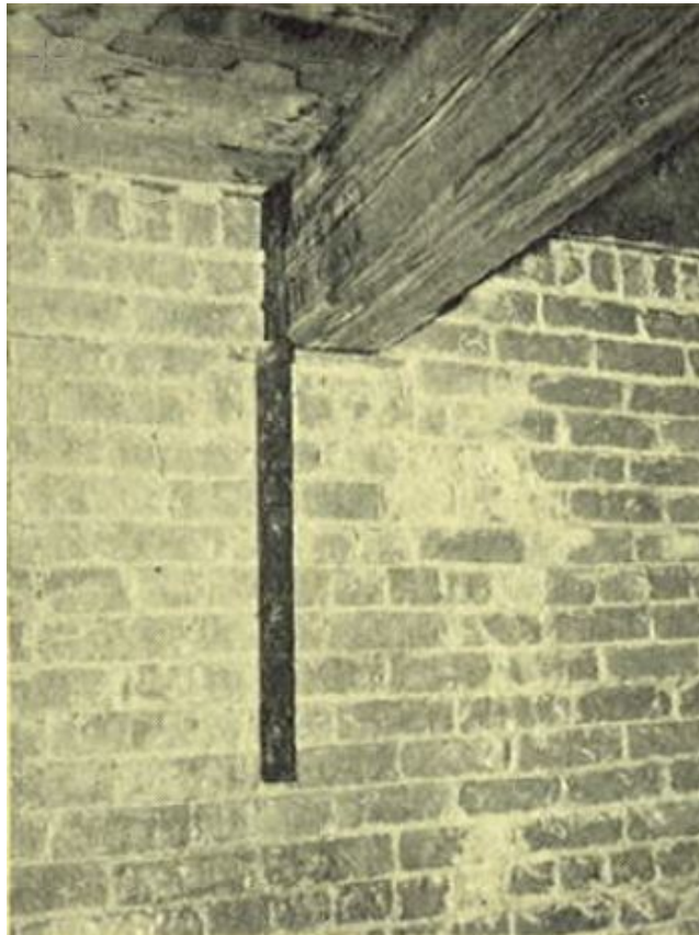
Fig. 3.1-7. Wood roof beam anchored with short steel straps and masonry anchors
