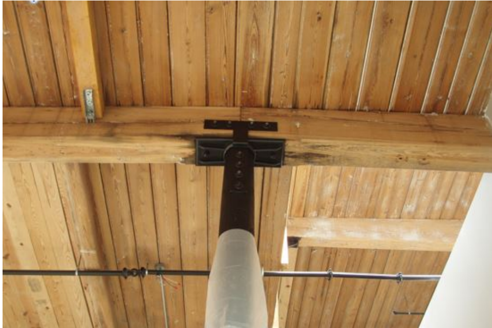
Fig. 3.1-8. Metal bracket added during renovation to anchor roof beam to the top of the building column (courtesy WinnResidential LP)
