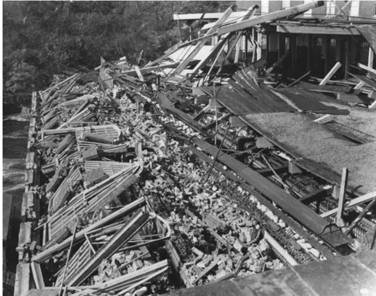
Fig. 3.2-2. Plank-on-timber textile mill damaged by the 1938 hurricane
