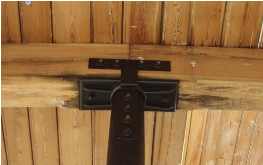
Fig. 3.1-8. Metal bracket added during renovation to anchor roof beam to the top of the building column (courtesy WinnResidential LP)
