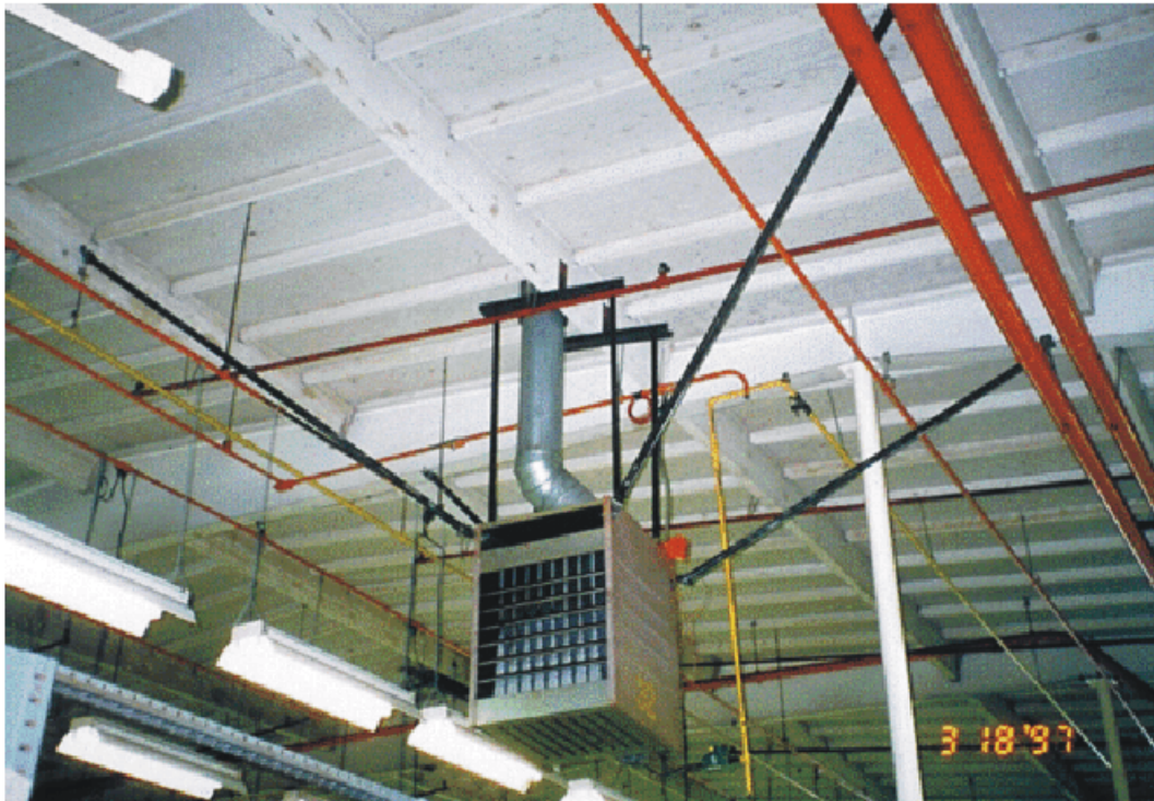
Fig. 2.3.1.1. Example of restraint for suspended space heaters
