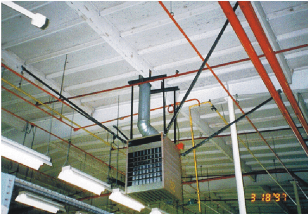
Fig. 2.3.1.1. Example of restraint for suspended space heaters
