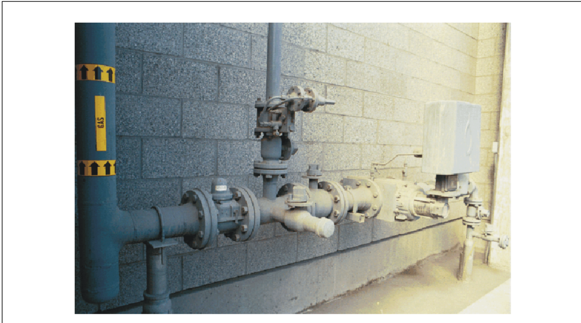
Fig. 2.3.5.4.1. Automatic integrated seismic gas shutoff valve (SGSV) installed in a fuel gas line downstream of pressure regulator
