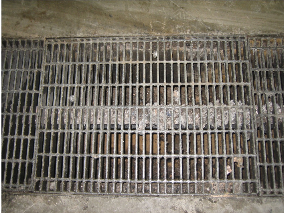
Fig. 9. An industrial-style drain grate with a free area of approximately 50%
