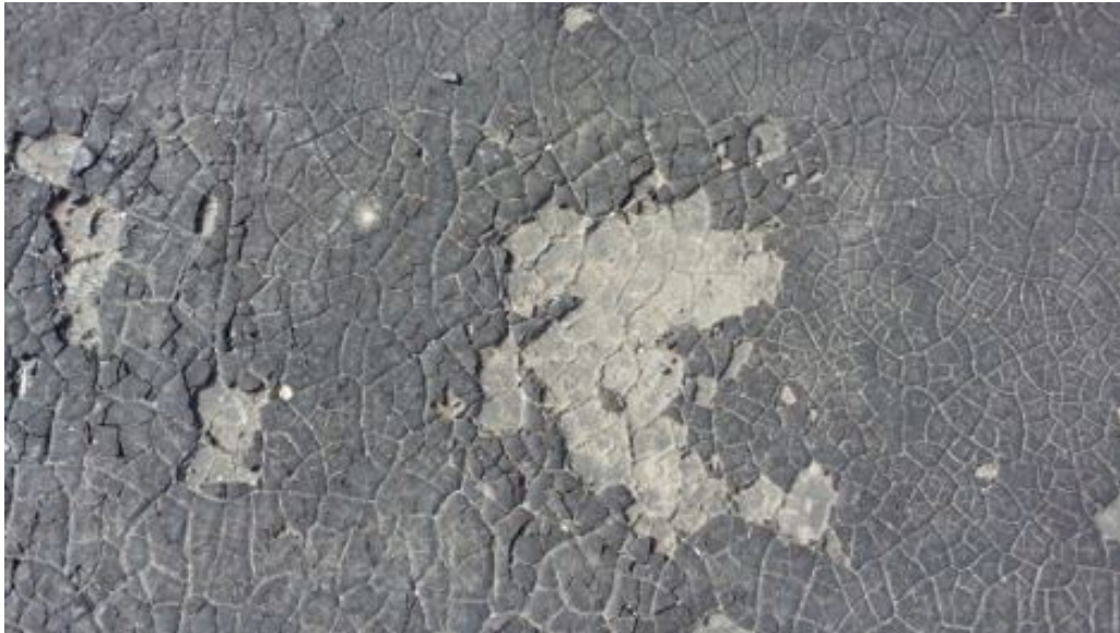
Fig. 1.1-1 Hail damage to 20-year-old "alligatored" built-up roof
