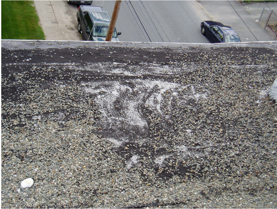
Fig. 3.1-10. Scrim showing where gravel is missing
