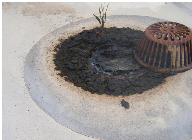
Fig. 3.1-2. Clogged roof drain
