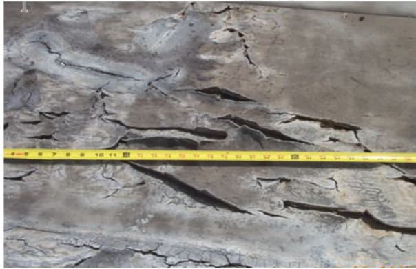
Fig. 3.1-6. Shrinkage and embrittlement of a thermoplastic single-ply roof with flaking of an incompatible asphaltic coating
