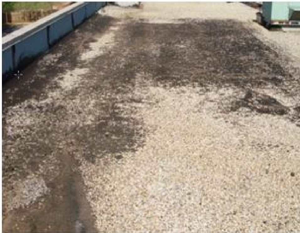
Fig. 3.1-9. Built-up roof with discolored area where water ponds (note exposed roof areas missing gravel)
