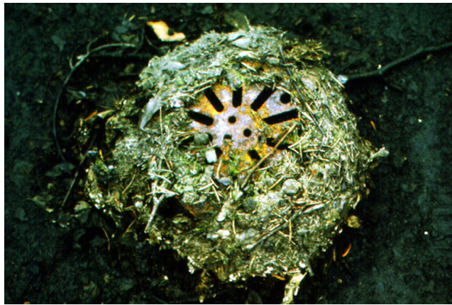
Fig. 3.1-1. Debris blocking roof drain
