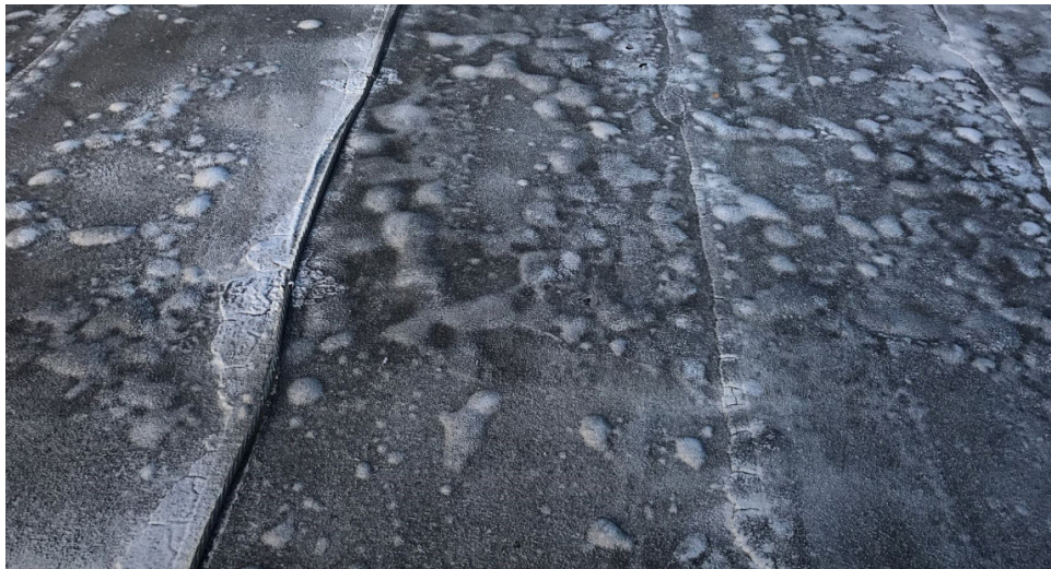
Fig. 3.1-8. Severe blistering of a built-up roof
