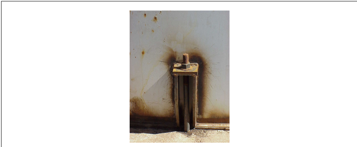
Fig. 27. Tank uplift anchorage chair
