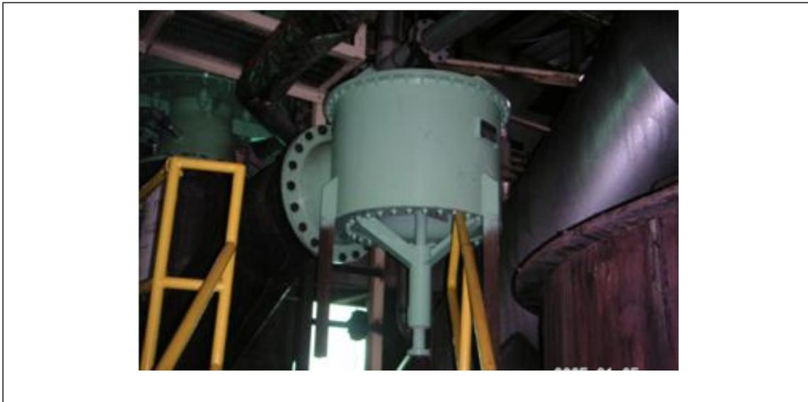
*Fig. 4. Eighteen in. (450 mm) diameter, weighted pallet vacuum relief valve (set pressure on order of inches of water [mm of water] with relief capacity on order of 20,000 scfm [566 m<sup>3</sup>/min] air)*
