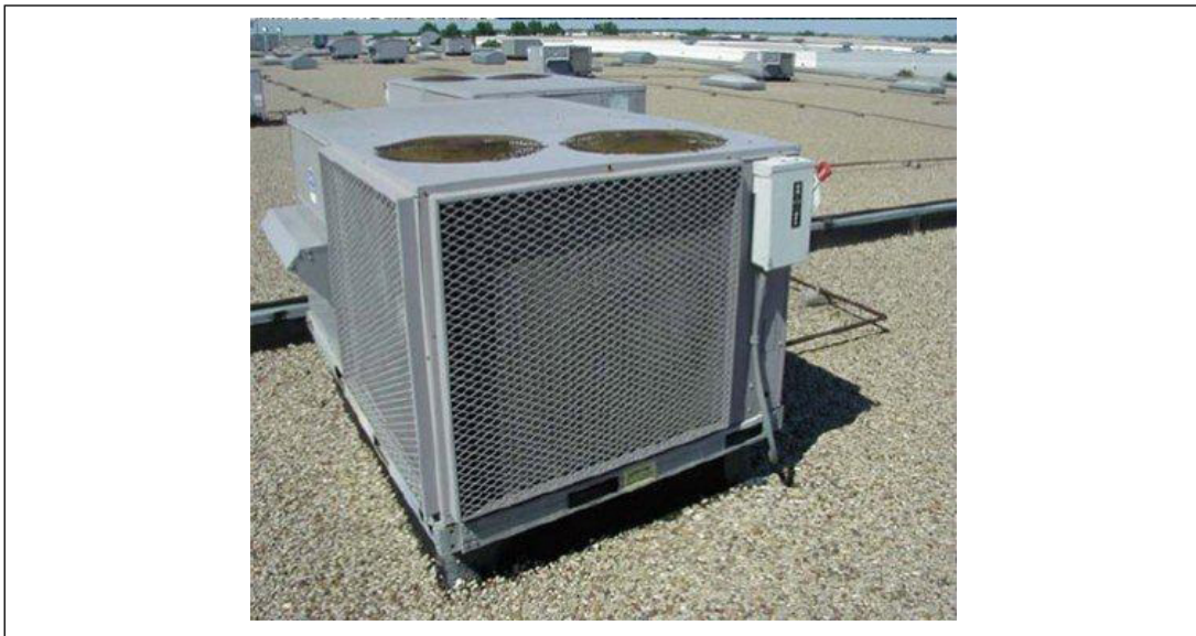
Fig. 3.3.1-2. HVAC unit with hail guard over condenser cooling fins at same location as hail damaged unit in Figure 3.3.1-1
