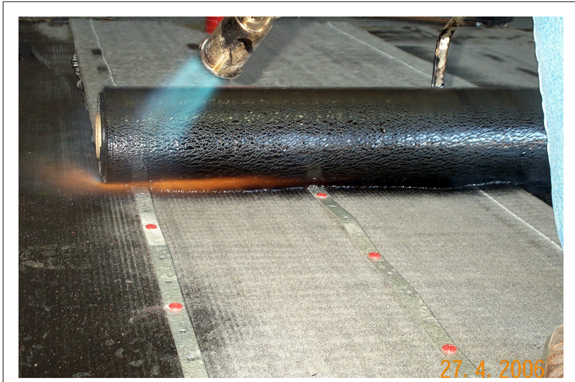
Fig. 1. Torch application of upper ply to a mechanically fastened base sheet — Note adhesive pooling at the leading edge of the roll. Also, screws and stress plates or batten bars are steel as they could come in contact with the torch flame. The screws in this figure are actually coated steel, not plastic.
