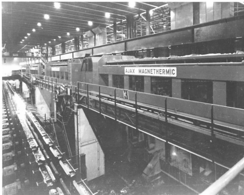
Fig. C.1-3. World's largest induction heating installation for heating steel slabs, showing discharge side of heaters and heated slab on conveyor to mill. (Ajax Magnethermic Corp.)
