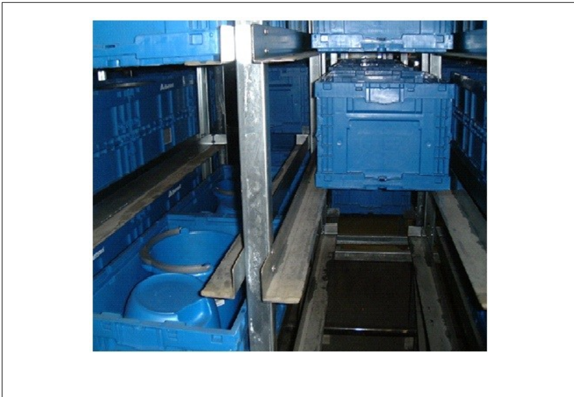
Fig. 3.1.1(b). Example of a mini-load type horizontal-loading ASRS
