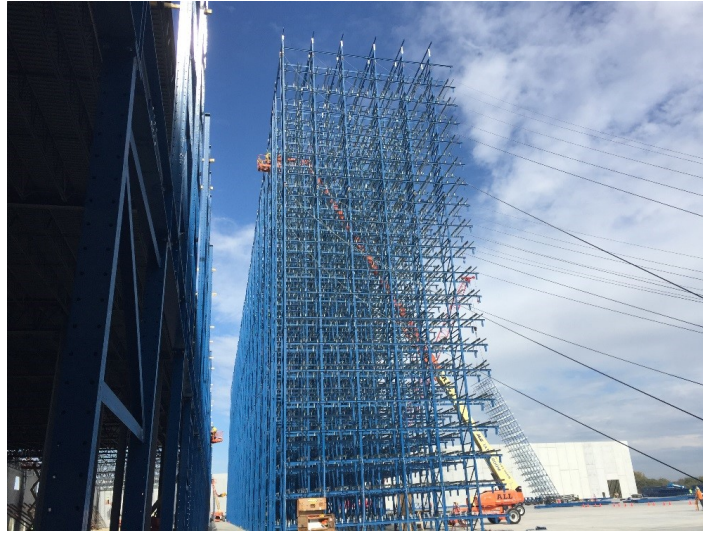
Fig. 59. Example of rack-supported ASRS storage arrangement
