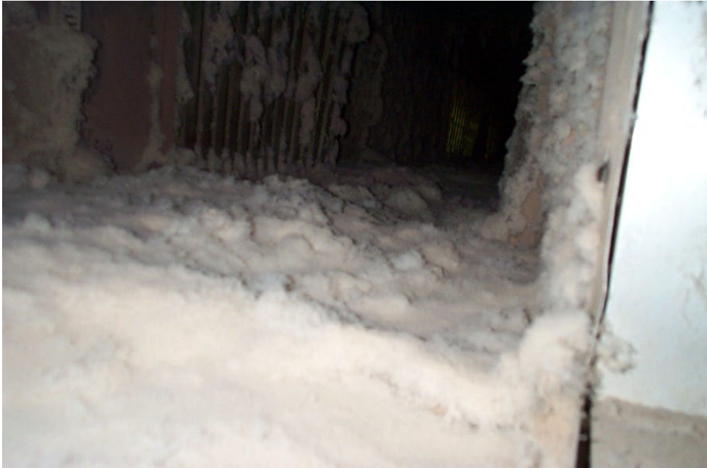
Fig. 3.3.9.2-3. Lint accumulation in supply air duct
