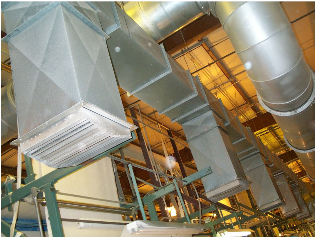
Fig. 3.3.9.2-4. Supply air ducts with vertical drops to registers
