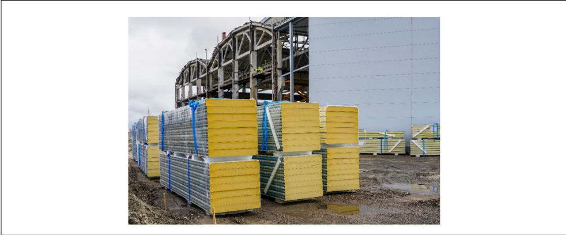
Fig. 3.2.1.1-1. Polyurethane foam core example (usually a yellow color)
