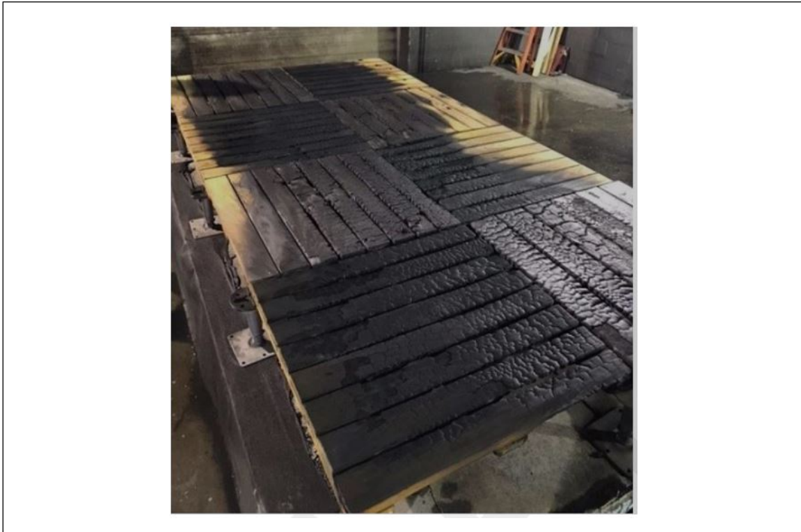
Fig. G.3-4. Ipe wood deck tiles prior to disassembly
