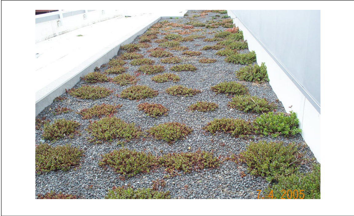
Fig. E-2. Extensive vegetative roof with sedums (courtesy of Genzyme Corp.)
