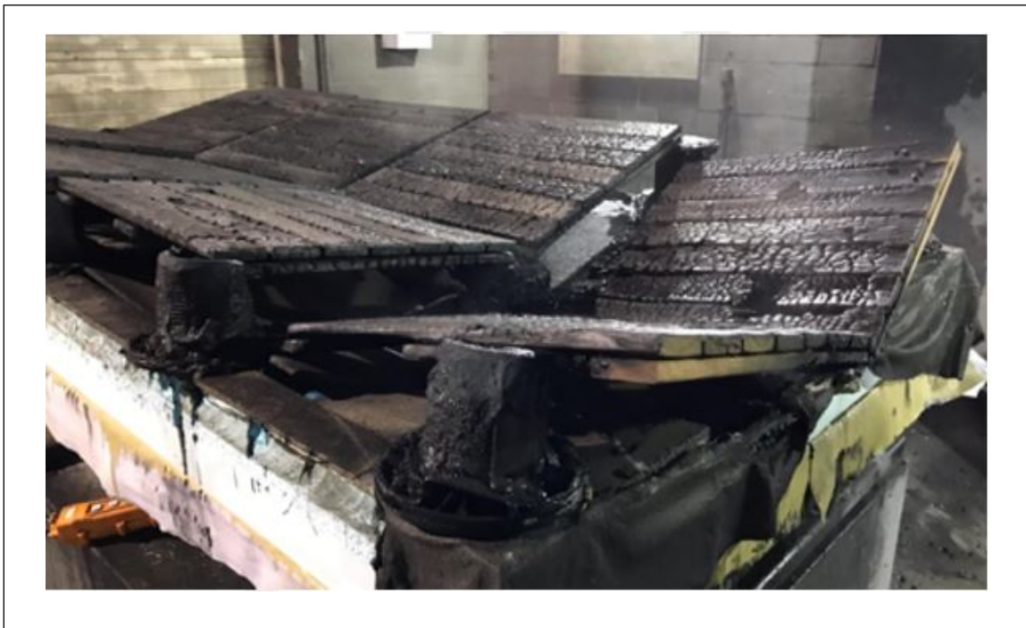
Fig. G.2-3. Aftermath of the fire test, prior to disassembly
